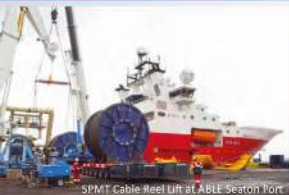
SPMT Cable Reel Lift at ABLE Seaton Port
