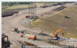
Excavators and MEWP at ABLE Seaton Port
