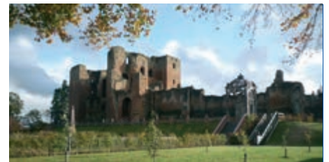
Steps and a disabled lift at Kenilworth Castle, Warwickshire.
