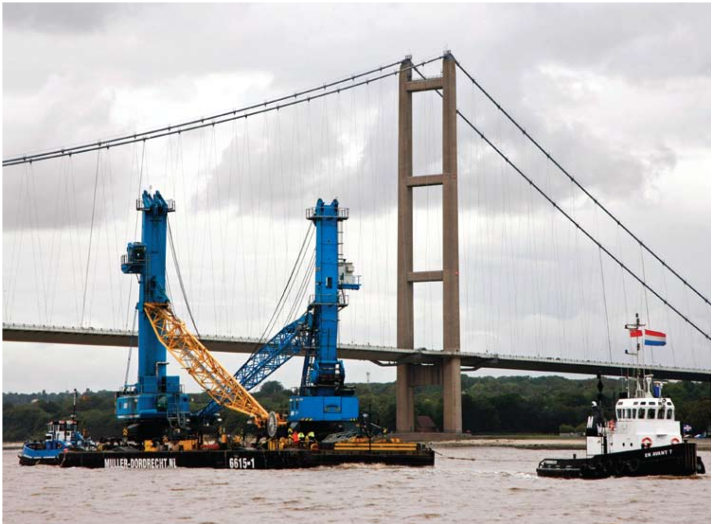
A barge, operated by Dutch-based Muller Dordrecht, at work on the Humber
