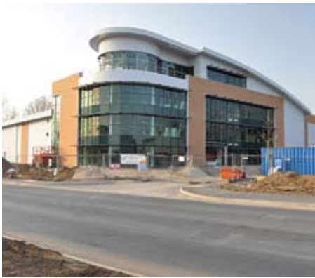
Work in progress on a new building for Allam Marine at Melton.
