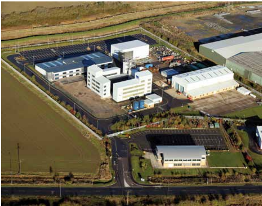
HCF CATCH site with the HETA building on the right.
