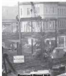
Prospect Street Hull
